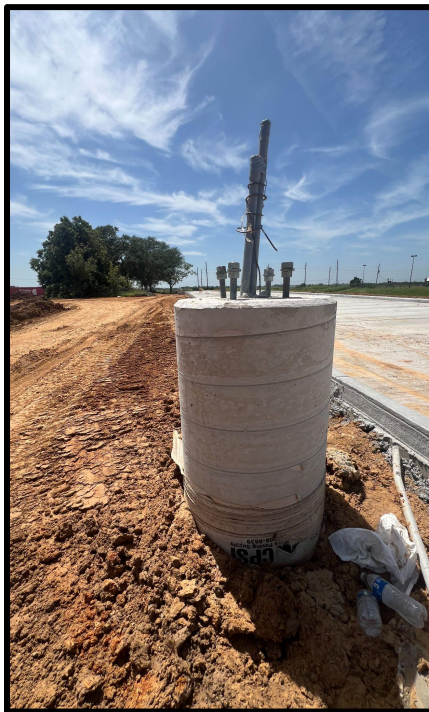
Road Paving and Light Pole Base
