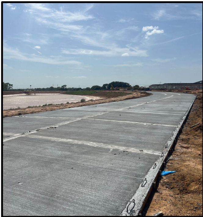
Road Paving and Light Pole Base
